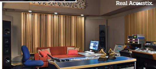
Rear diffusers and open ceiling construction help create a reflection-free zone. Inset: Behind the tape machines and racks are FlutterX panels from Real Acoustix.
